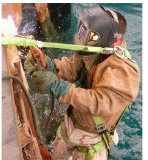
SW2 Eberly welding in the OPLATS
